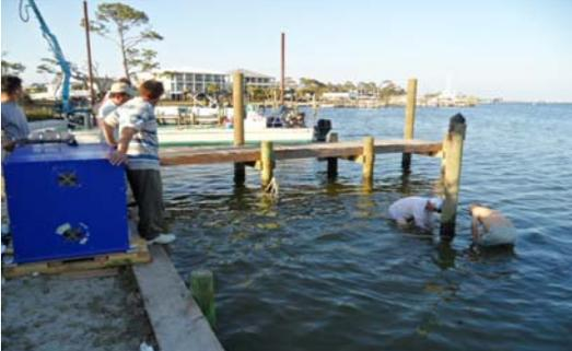
Additionally, the ionizer injects oxygen into the water which improves the cleaning aspects of the system. A standard model will raise DO in the immediate area to as high as 25 parts-per-million (PPM) and in the area of 18-20 PPM at a distance of a quarter mile. DO readings around 7 PPM are considered the benchmark. High levels of DO allow aerobic bacteria in the sand to thrive, enabling it to deal with any organic or inorganic pollutants.
